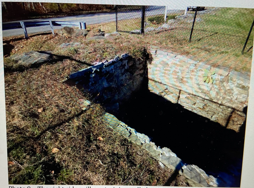
Photo 9 – The right side spillway training wall, the upper mortared section of which is in good condition.
