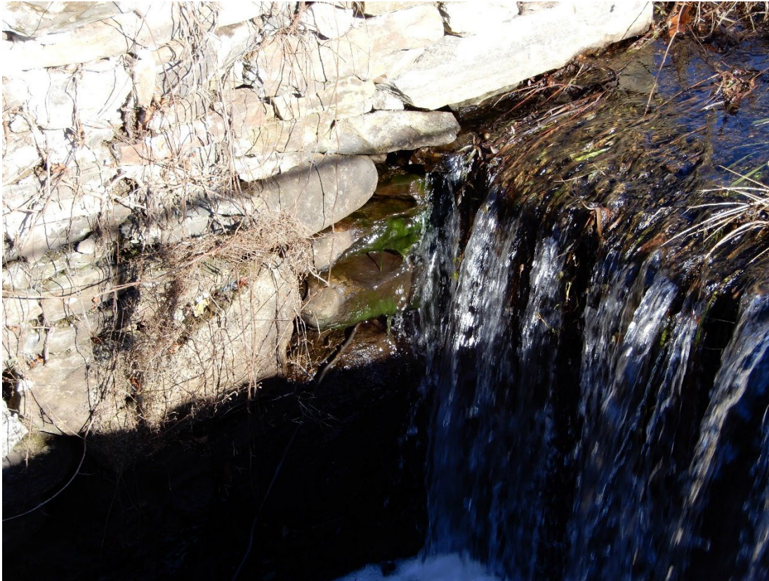
Photo 11 – Another view of the same right side wall, showing seepage through the open stone area directly adjacent to the spillway weir section.
