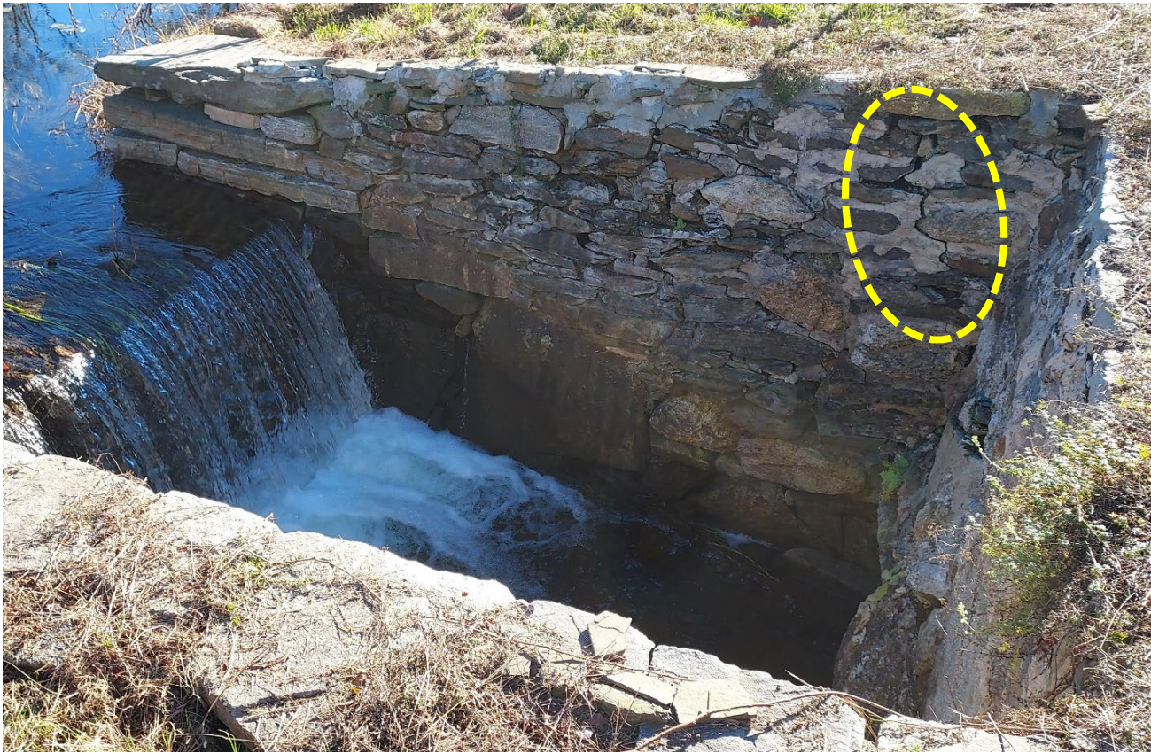
Photo 5 – The left side upstream training wall, highlighting a slightly diagonal vertical crack in the mortared masonry wall.
