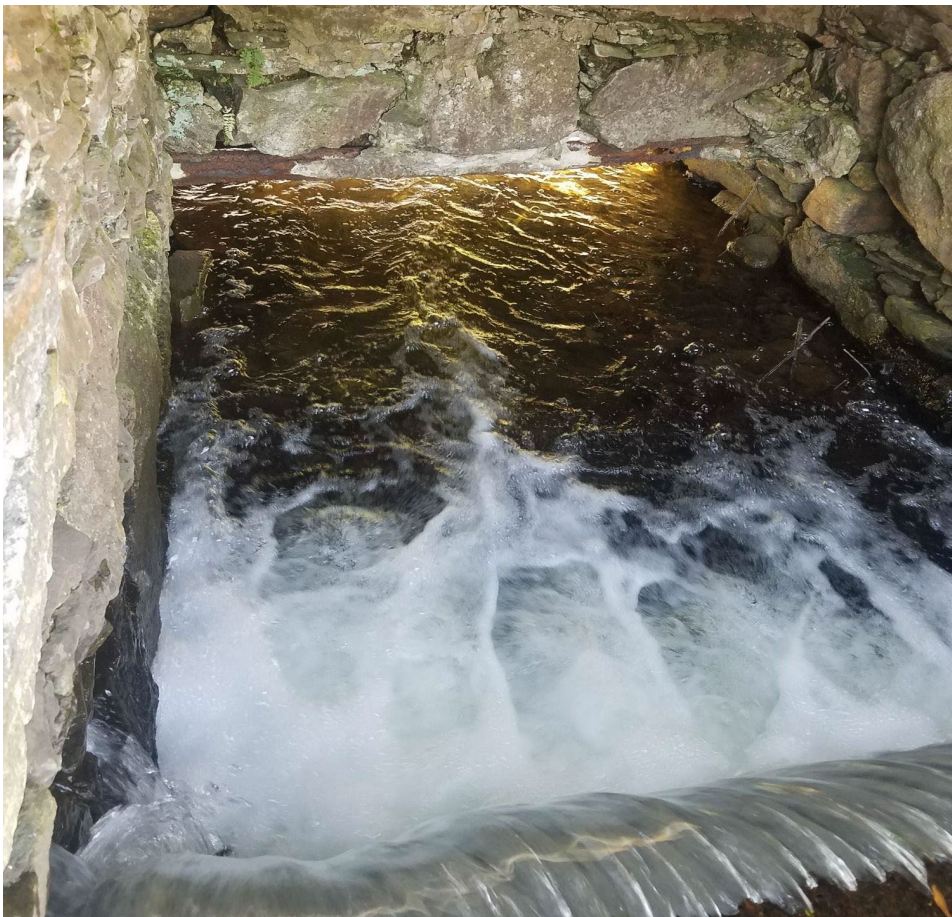
Photo 11 – Another view of the same right side wall, showing seepage through the open stone area directly adjacent to the spillway weir section.
