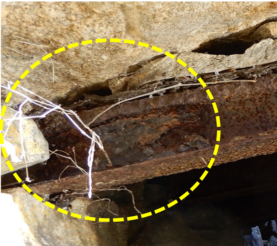
Photo 7 – A closeup of the right side downstream rail section, showing advanced corrosion and loss of section at the supporting end at the left side of the photo. Other underlying rail supports, although difficult to photograph, are in similar condition.
