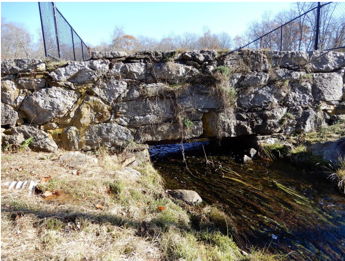
Photo 2 – The spillway area as seen from a downstream perspective.
