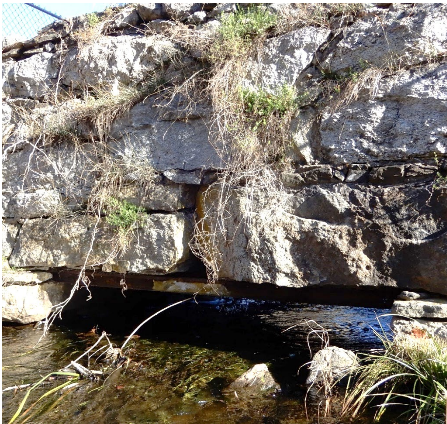
Photo 5 – The left side upstream training wall, highlighting a slightly diagonal vertical crack in the mortared masonry wall.
