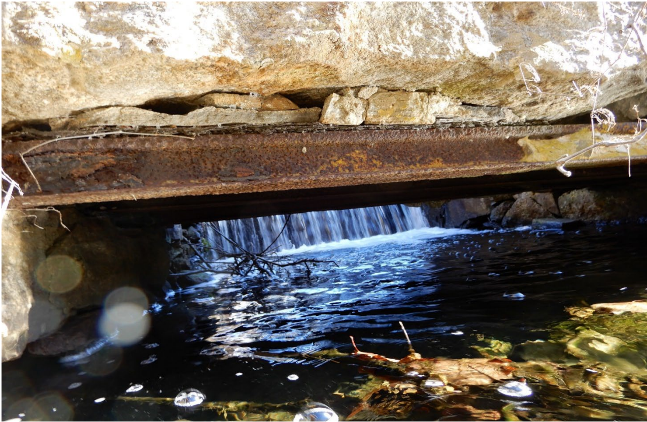
Photo 7 – A closeup of the right side downstream rail section, showing advanced corrosion and loss of section at the supporting end at the left side of the photo. Other underlying rail supports, although difficult to photograph, are in similar condition.
